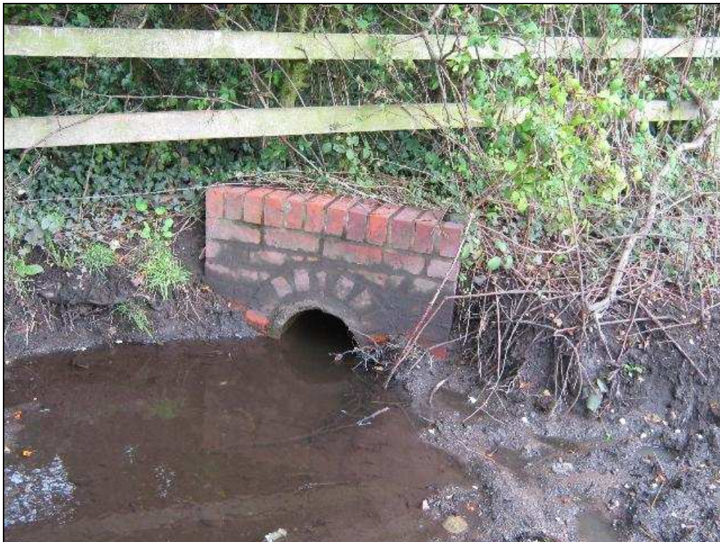
Plate 4: Stream B showing the culvert at the eastern end
