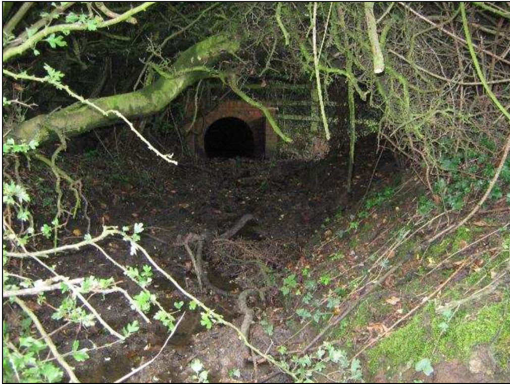
Plate 9: Stream D – Showing heavily canopied culvert at eastern end
