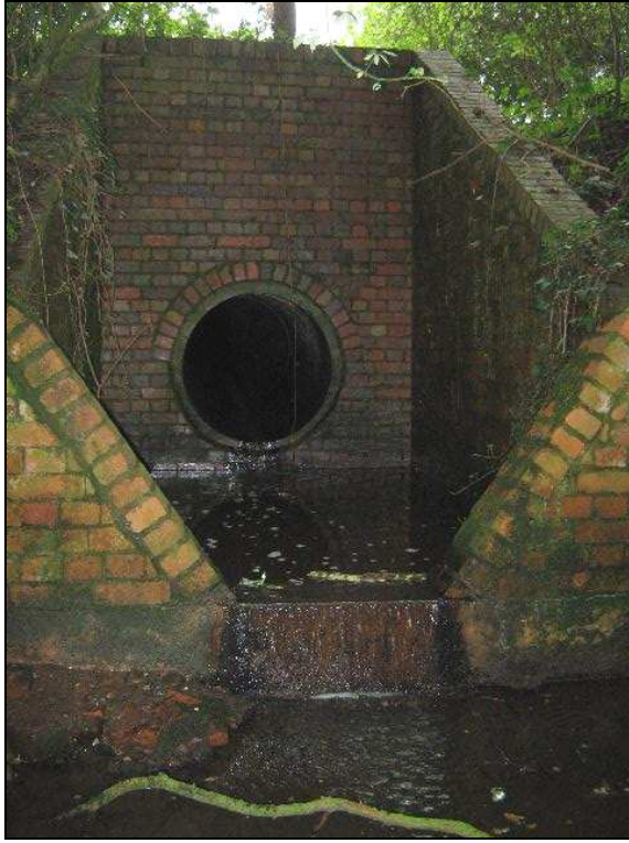
Plate 5: Stream C- culvert at stream entrance
